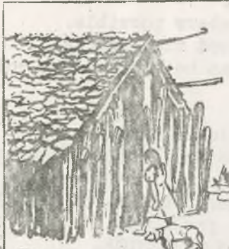
THE HUTS OF THE OTOMI INDIANS OF MEXICO, HAVE WALLS MADE FROM THE ORGAN CACTUS AND A ROOF OF CACTUS LEAVES
