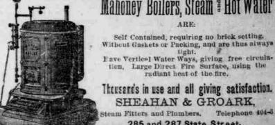
Mahoney Boilers, Steam & Hot Water Self Contained, requiring no brick setting. Without Gaskets or Packing, and are thus always
