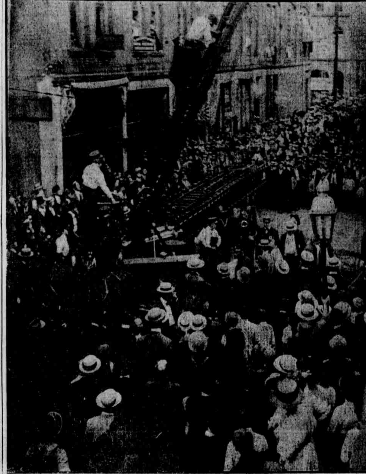
Fireman Guiding Rescued Lineman Down Aerial Ladder.
